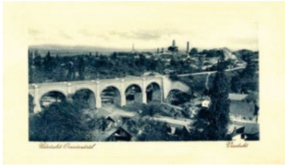
Figure 8: Viaduct, Baziaş area [6]
